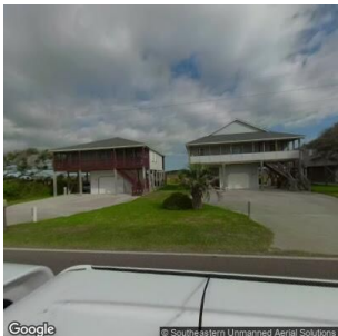
© Google © Southeastern Unmanned Aerial Solutions
