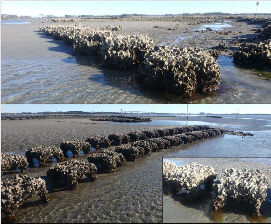
Figure 6. Examples of oyster growth on stacked Oyster Catcher™ Tables (top); rows of single Oyster Catcher™ Tables (bottom) and close-up of oyster growth on Tables (bottom insert) 18 months after deployment in North Carolina.
