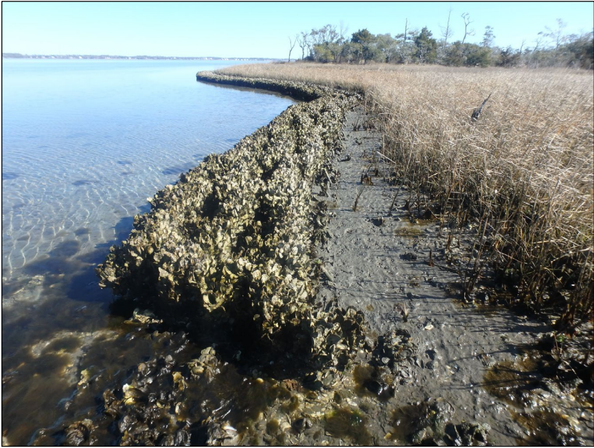
Figure 7. Oyster Catcher™ reef (185 ft) at the NC Aquarium at Pine Knoll Shores. Sill constructed April 2019; picture date February 10, 2022. Note that plant growth during spring and summer 2022 has expanded this saltmarsh to the back edge of the sill.
