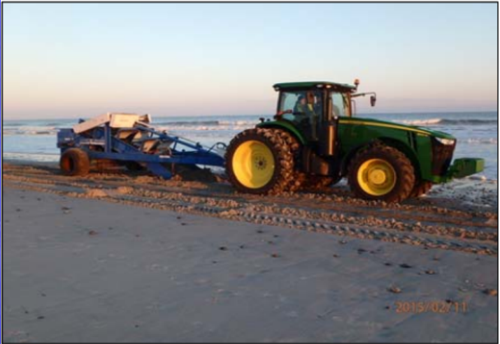
Photo 2. The rock picker was dragged behind a tractor along the beach fill area to remove rocks between Sta. 755+00 to 750+00.
