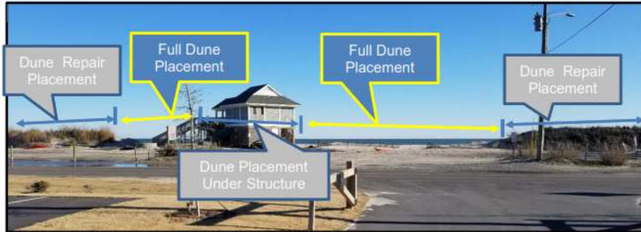
Figure 1: Dune Material Placement (photo taken February 3, 2021).
