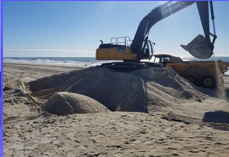
Transfer from Dump Trucks to All-Wheel Drive Beach Dump Trucks
