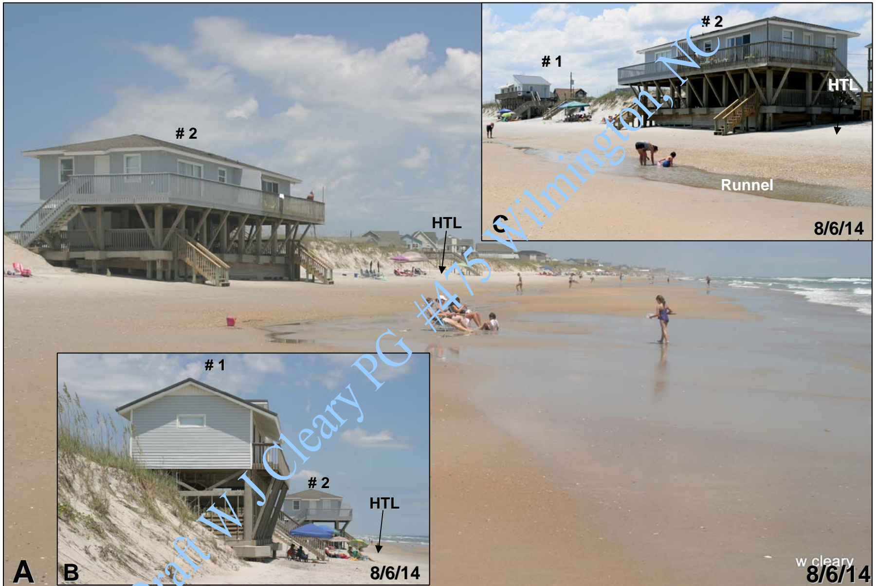
Figure 35. The NTE shoreline during a rising Spring tide on 8/6/14. A. Northerly view of home #2 perched along the dune. Note position of the HT swash line. B. Northerly view of homes #1 and #2 along dune line. High tide swash line lies near base of dune. C. Southerly view of homes # 1 and # 2. Despite numerous storms that eroded the dunes, the HTL position has changed little during the past 25 years.
