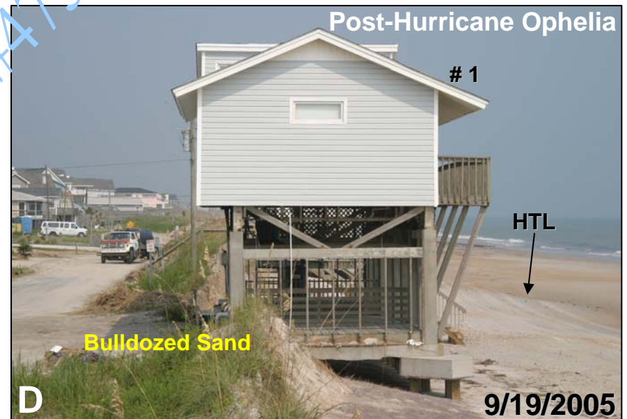
Figure 34. Shoreline changes along southern portion of North Topsail Beach between July 2002 and September 2005. A. Northerly view (7/7/02) of homes perched along artificial dune line. Note pilings are exposed near HT swash line. B. Aerial view (9/20/05) depicting the minimal impact of Hurricane Ophelia. Note scarped dune line and position HT line. C. Northerly view (9/19/05) of homes with exposed foundation slabs. Note gravel strewn foreshore. Coarse shell and lithic fragments were derived from residual sediment accumulations that mantled hardbottoms. Extensive high-marsh peat exposures front much of this area. D. Northerly view of home # 1 along restored dune line. Despite numerous tropical storms, hurricanes and extra-tropical storms, some of which produced surges that inundated the island, the HTL position has changed very little since 1952. Erosion rates in this vicinity range from 0.6 to 0.7 ft/yr. See Figure 32 A.
